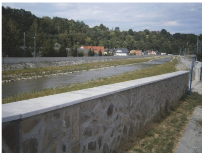
Fig. 3. Realized concrete flood protection walls in the middle part of Bardejov town (phase I.) (Šoltész et al., 2018b).
