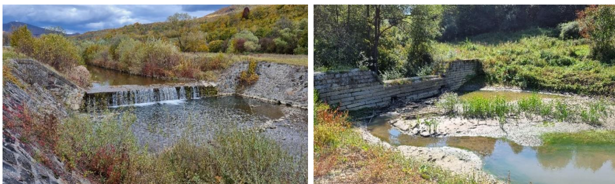
Fig. 3. Existing measures on the Zbojský stream (a) and on the Tapovec stream (b).
