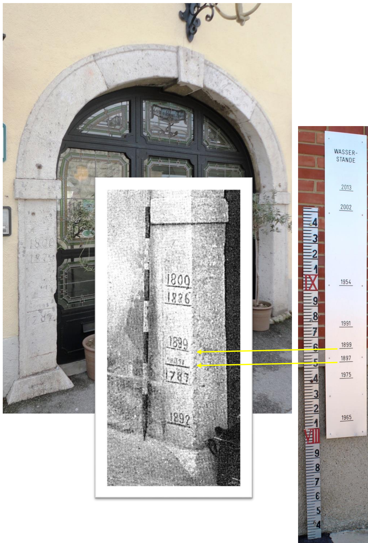
Fig. 2.2h The Danube flood marks, Hainburg. (cutout photo from Lauda et al. (1908) (big photo: Pekárová, 2011; Miklánek, 2019).
